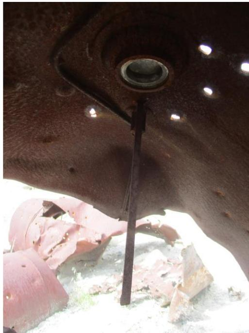
Interior of the fuel tank, with filler cap at top
