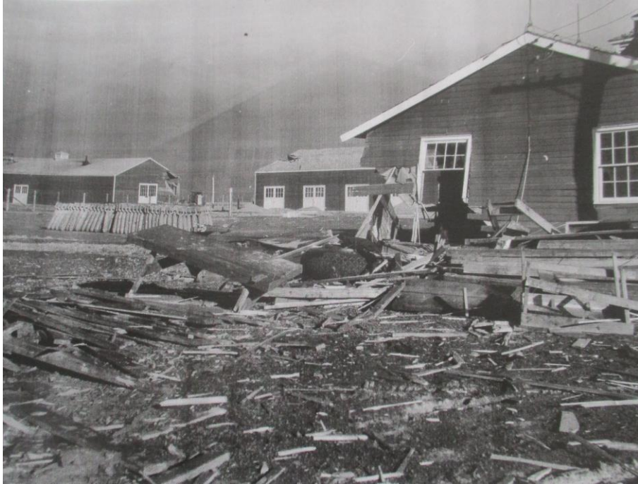
Damage to the three buildings is shown in this photo. The photographer was standing with his back to the aircraft wreckage. The closest structure was torn down after the accident. (Courtesy of Craig Fuller/AAIR)
